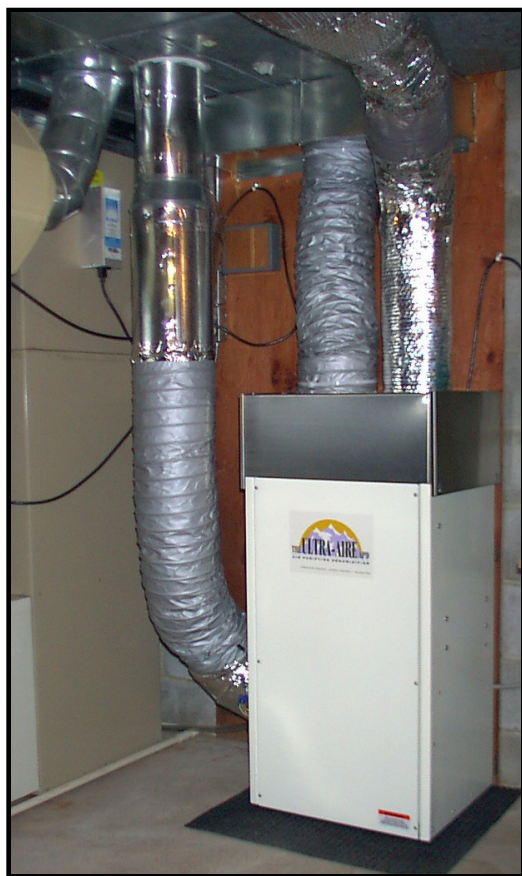
A whole house ducted dehumidifier delivers the ultimate in comfort and healthy indoor air
